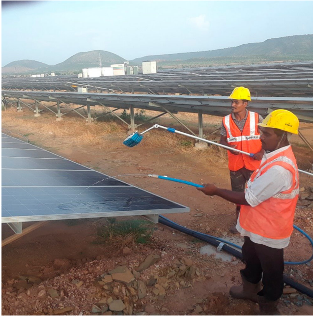
Figure 6. Laborers cleaning the solar panels at the Kurnool Solar Park. (Photo: Ryan Stock).
