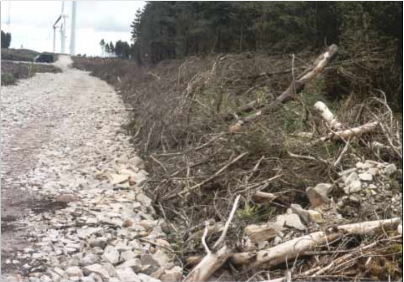
Plate 7: A supposedly ‘floating’ road actually sinking rapidly and likely to flood when heavy rain falls.
