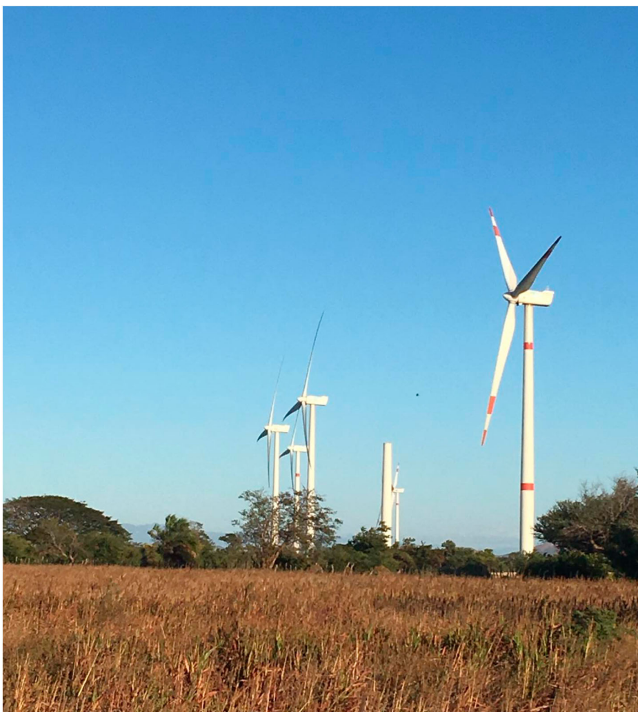
Figure 3. DEMEX wind turbines, Unión Hidalgo. Source: Alexander Dunlap.
