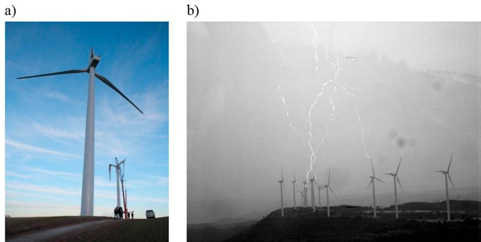
**Figure 1.** (a) Example of lightning damage to blades of two wind turbines due to a winter storm in the northeast of Spain in 2009. (b) Integrated frames of a high-speed video (available in the supporting information). Three upward positive lightning leaders progressed from rotating wind turbines. Also three wind turbines showed short-lived aborted leaders. The event occurred in the same wind farm as in Figure 1a on 1 July 2012.
