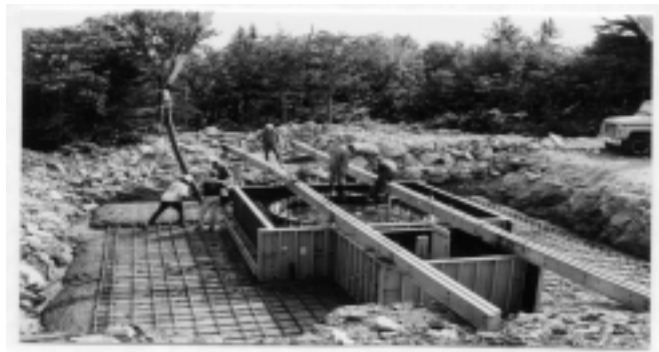
Figure 6-3 Foundation Construction at the GMP Project Site
