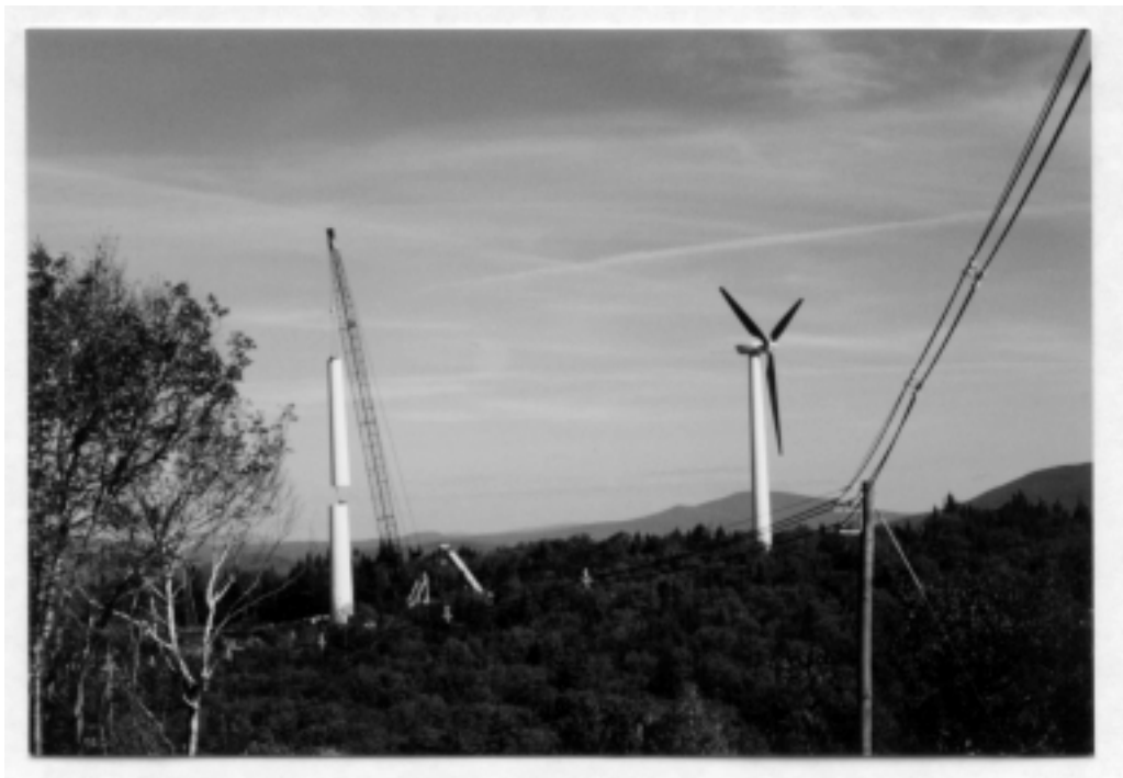
Figure 6-5 Installation of a Top Tower Section
