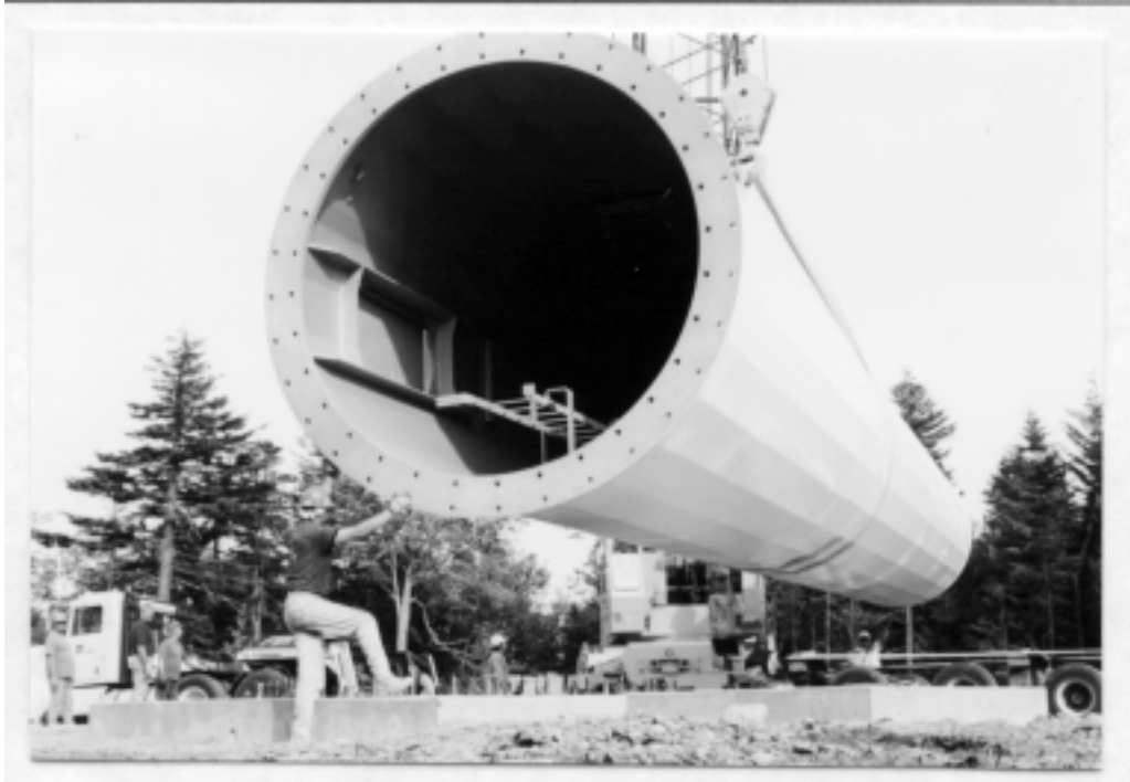
Figure 6-4 Off Loading a Bottom Tower Section at the Site
