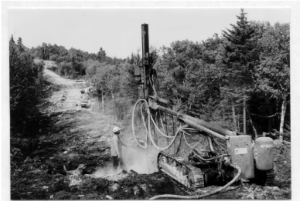
Figure 6-1 Access Road at Site Under Construction
