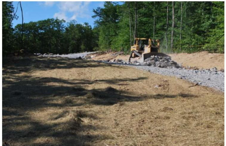
J.A. McDonald bulldozer setting the rough grade for the service road. Erosion control measures are undertaken in parallel with construction to ensure minimal impacts from run-off.
