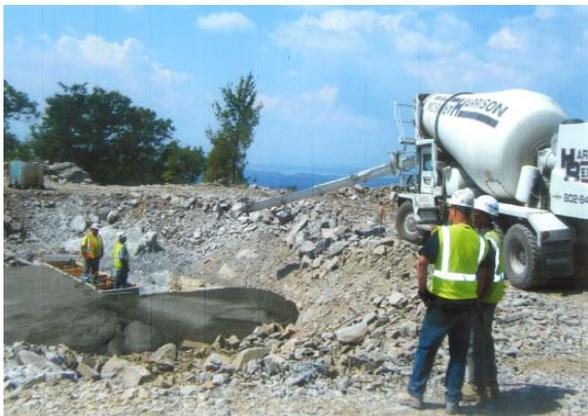
First concrete footing is poured for turbine 3 on July 25<sup>th</sup>.
