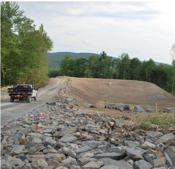
A newly completed storm water retention pond midway up the service road is the largest of four reservoirs constructed.
