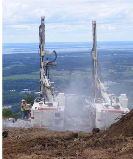
Drilling rigs work to prepare a wind turbine foundation site at the top of the mountain with Lake Champlain in the background.
