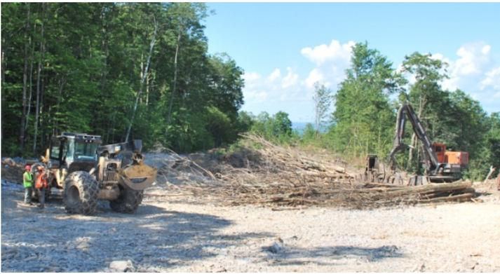
Site clearing work for the service road to the northern two turbine sites is made ready for excavation. Clearing work was done by Doug Edwards Timber Harvesting from Cambridge Vermont.
