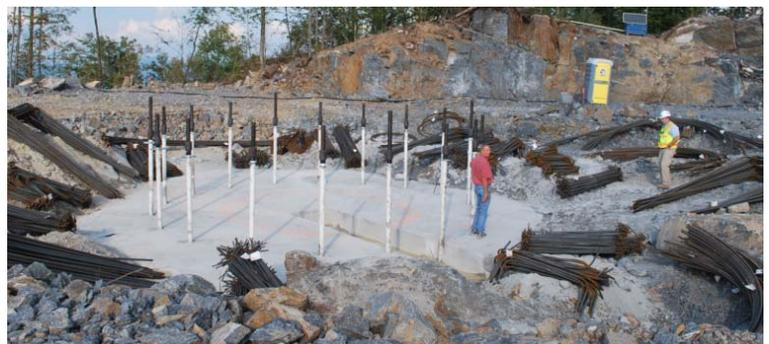
Rock anchor rods protrude approximately 8 feet from the footing for a turbine foundation. Rebar will be installed inside the ring of anchor rods before the concrete foundation is poured nearly to within 1 foot of the top of the rods.
