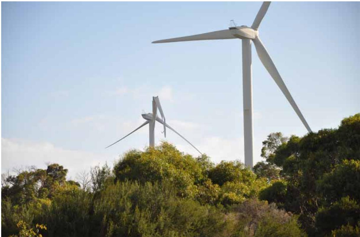
Blade failure in March 2012 approximately 6 years after it was commissioned. Blade failures are common worldwide.
