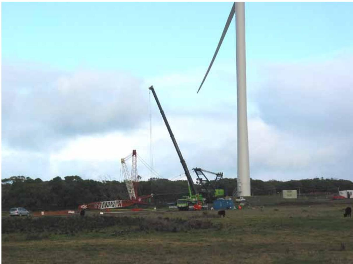
Replacing the rotor bearing on a turbine at the six turbine wind farm in 2007 approximately one year after it was constructed.
