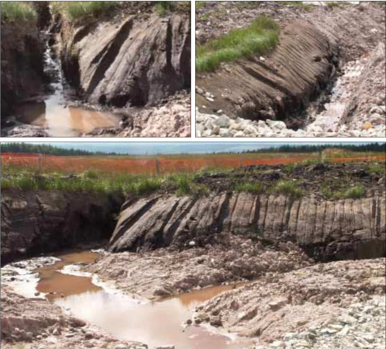
Plate 7. Top left: the drainage channel for a turbine base; the boulder clay under the peat is clearly visible. Top right: in several places on the site, boulder clay exposed in this manner is already eroding, leaving peat high and dry. Above: the drainage arrangement for turbine bases. Silt in the stagnant pools is to be trapped by silt beds (see pages 14 and 29).
