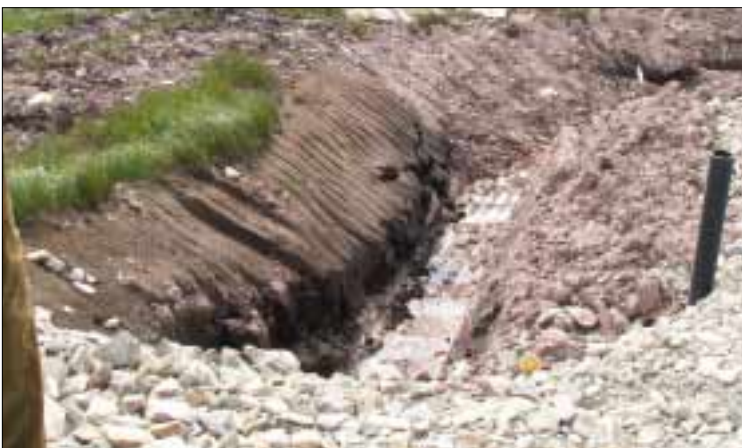
Plate 10, above left: The surround for a turbine base showing boulder clay under the peat.
