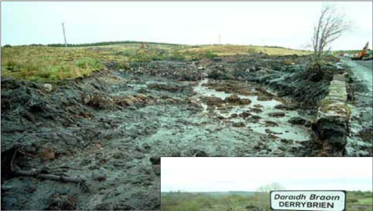
Plate 1, above: Peat from the bogslide, by now a thixotropic slurry, pressing on the Flaggy Bridge just east of Derrybrien. The bridge was closed for several days amid fears that it would collapse. The watercourse is normally three to four metres below the road level.
