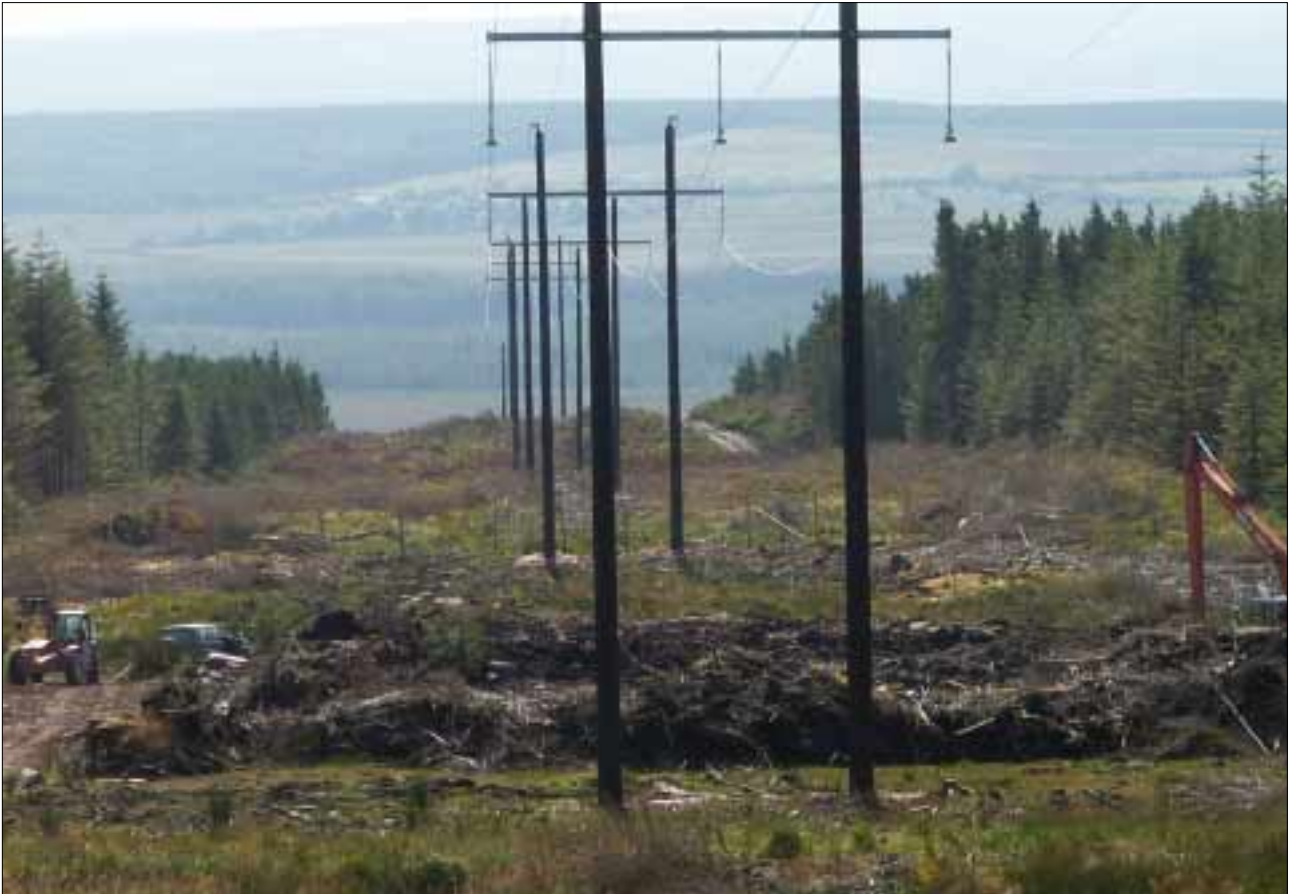
Plate 19: One of the peat lagoons discussed on page 13. The watercourse polluted by the bogslide runs right to left behind the mechanical digger in the left foreground. Peat still in the watercourse, now restrained by a bund, was being lifted into the peat-walled lagoon visible in the foreground. (The power line is the site's 110kV link to the grid.)
