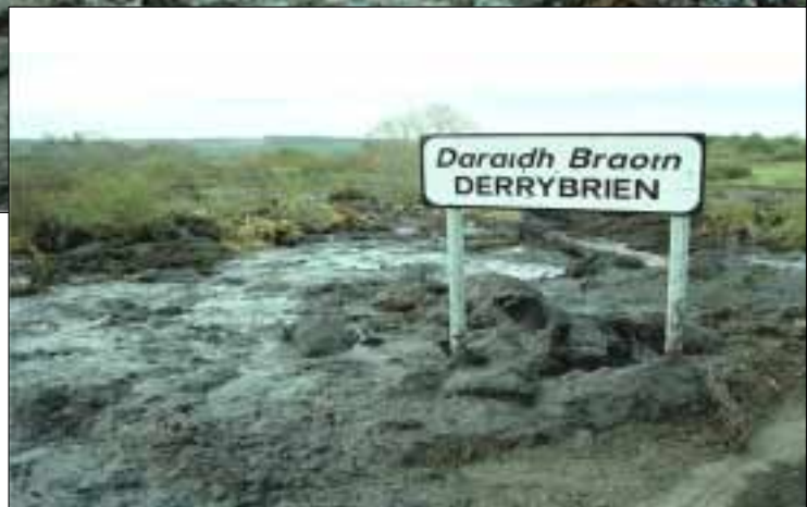
Plate 1, above: Peat from the bogslide, by now a thixotropic slurry, pressing on the Flaggy Bridge just east of Derrybrien. The bridge was closed for several days amid fears that it would collapse. The watercourse is normally three to four metres below the road level.
