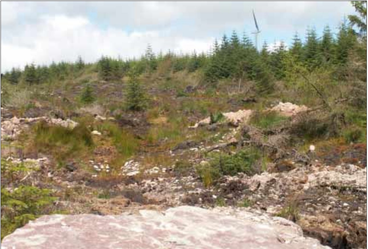
Plate 16, above: Looking up from a causeway built across the path of the slide to stop peat that is no longer there from sliding again. Note the drop in ground level compared to the surrounding afforestation.
