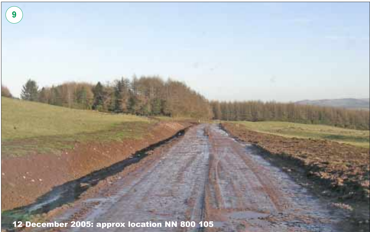
12 December 2005: approx location NN 800 105 Looking east from point 9. The design of the road is such that water is collected on the upslope side and runs via a deep ditch (with no silt barriers) into a natural water course. No effort was made to release water at intervals onto the downside grass and bracken area which would have acted as a natural silt trap. The results are shown below.
