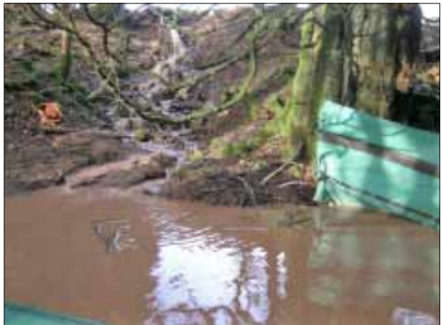
Point 13: the road at this point is barely 20 metres from the Bullie Burn. The top picture shows silted water being discharged from the road through the intervening wood into a silt catching system (middle and bottom). At least on the day these pictures were taken, it was manifestly failing. All this water ends up in the Bullie Burn.
