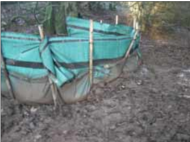
Point 13: the road at this point is barely 20 metres from the Bullie Burn. The top picture shows silted water being discharged from the road through the intervening wood into a silt catching system (middle and bottom). At least on the day these pictures were taken, it was manifestly failing. All this water ends up in the Bullie Burn.
