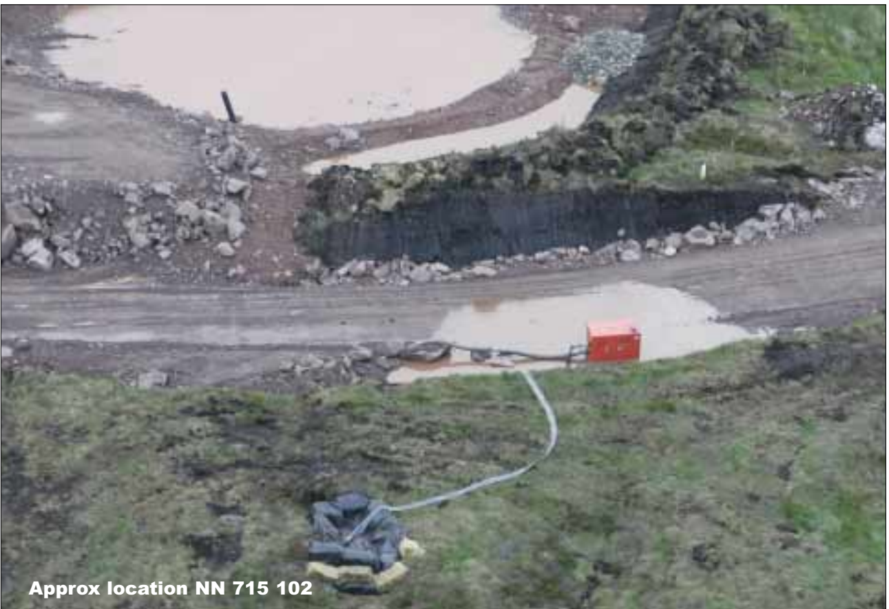
The excavation for a turbine base and the adjacent access road. The red box is a pump moving turbid water into a terram dam with small bales intended to catch silt downstream.
