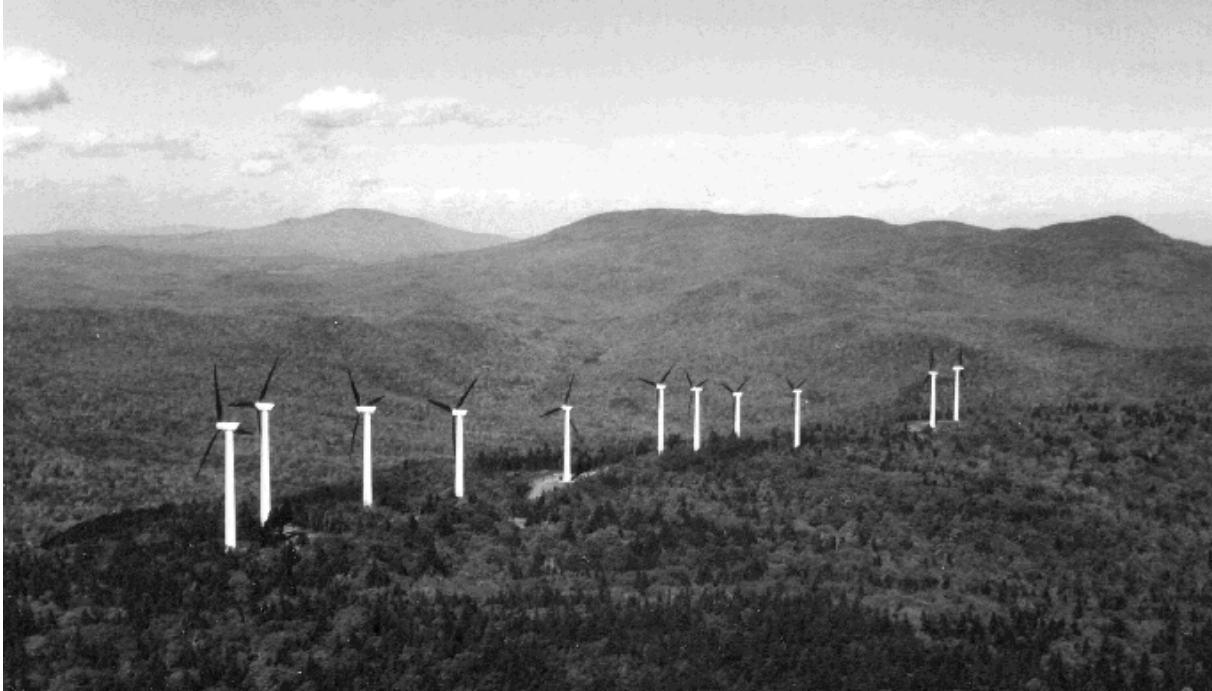
Figure 1-1 Photograph of the GMP Wind Power Plant
