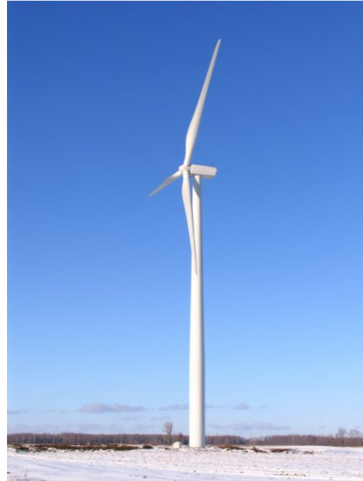
Richmond Road turbine, post construction 2006
